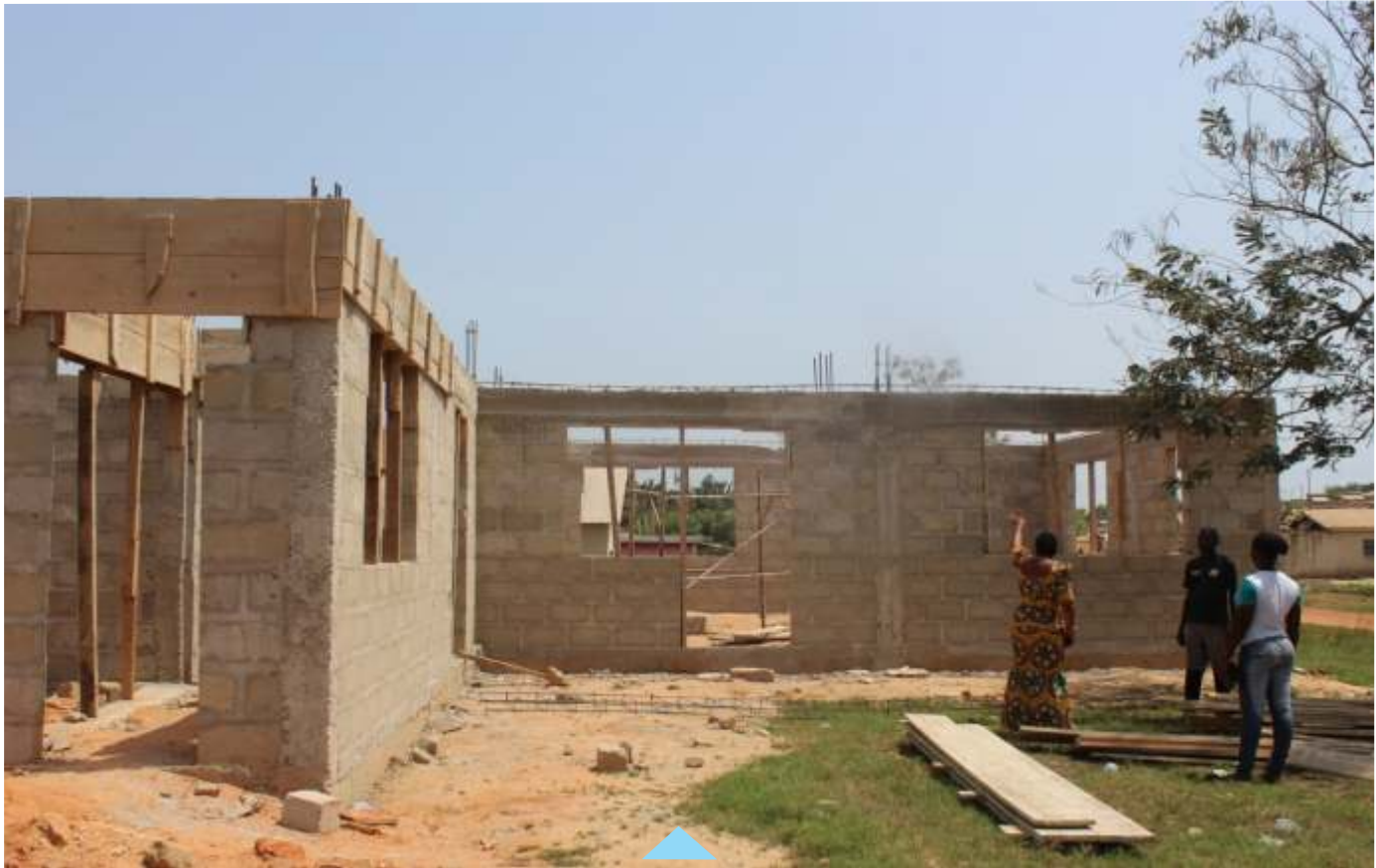
Community Health/Counseling center under construction at Nyankrom
