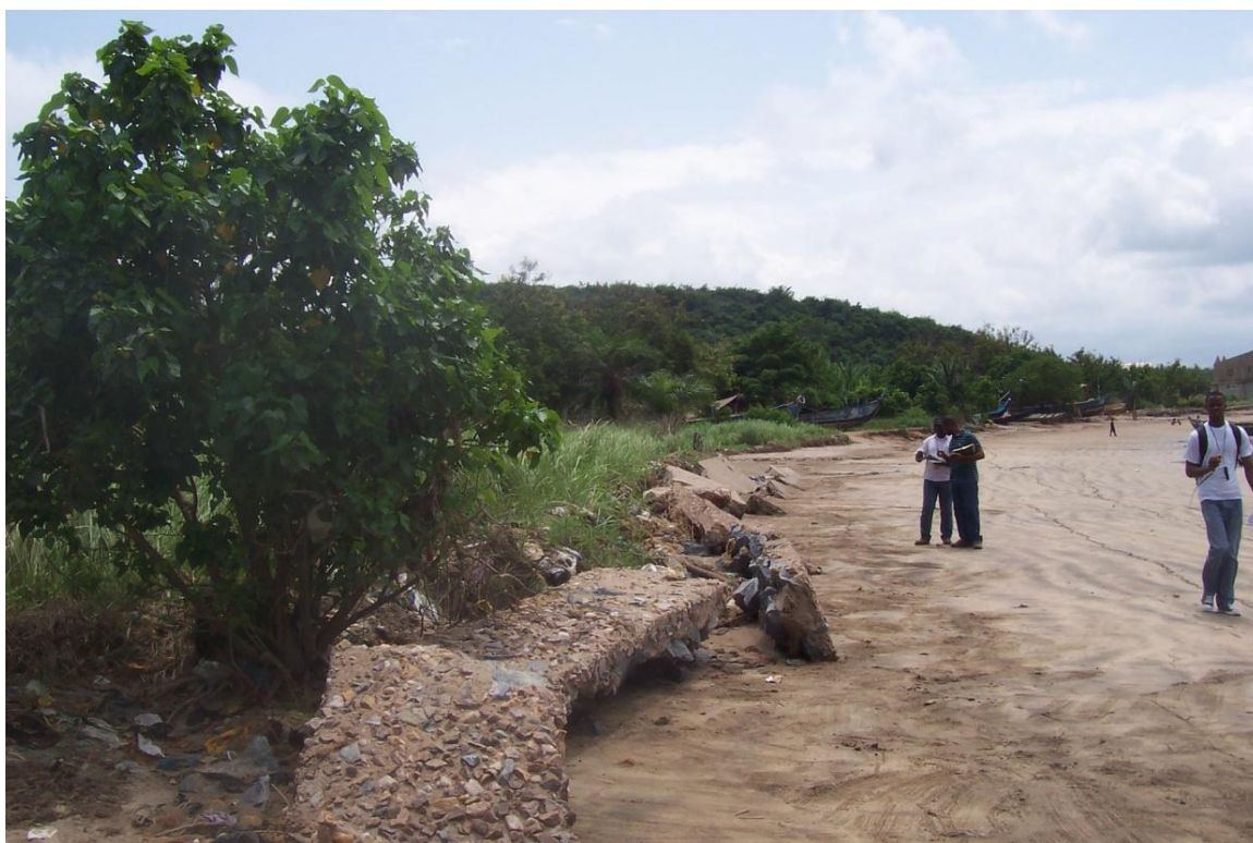
Plate 8 i: Shama Collapsed Sea Defence Wall
