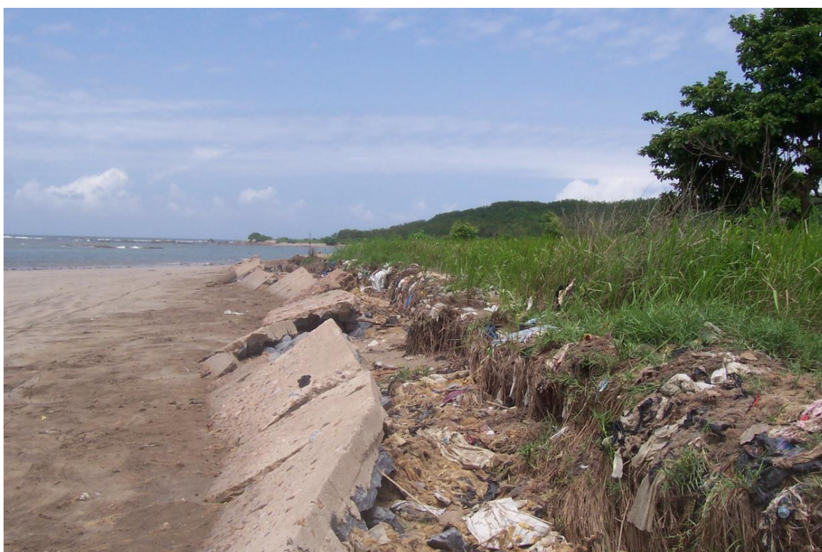
Plate 8 ii: Shama Collapsed Sea Defence Wall
