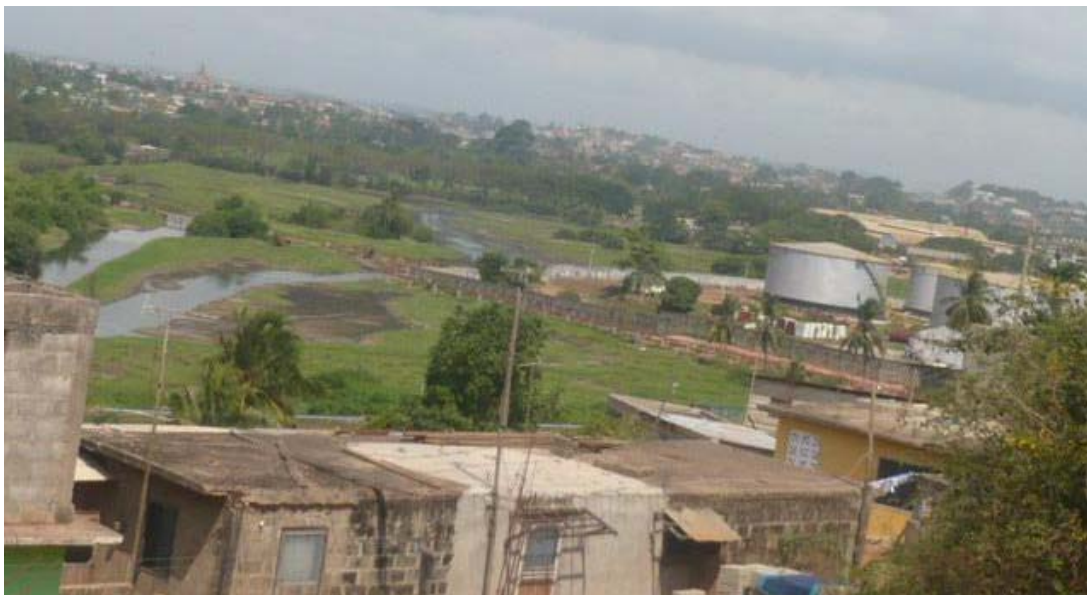
Figure 10: Aerial view of developments in a wetland area
