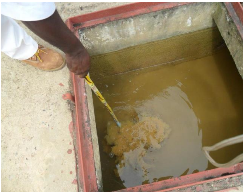
Fig. 6: excessive dirt builds up in sediment tank at GWCL, hence requiring constant dislodging
